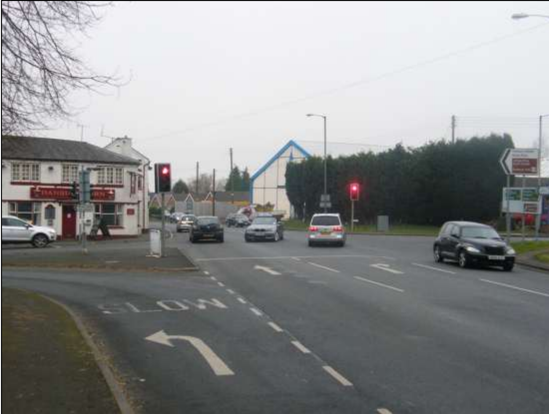
Photo 1: Looking NW at Hanbury Turn crossroads layout
