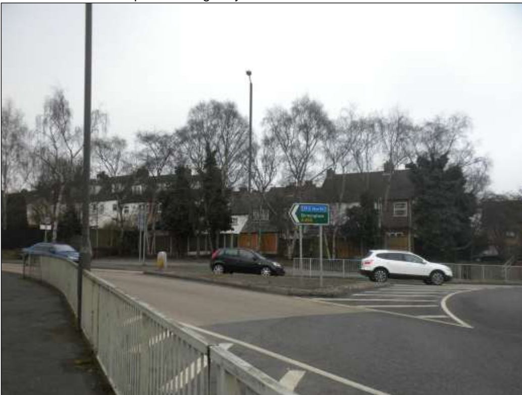
Photo 9 – View of part of the AQMA at Coventry Street island at the junction with Coventry Street, note closeness of receptors to Ring Way.
