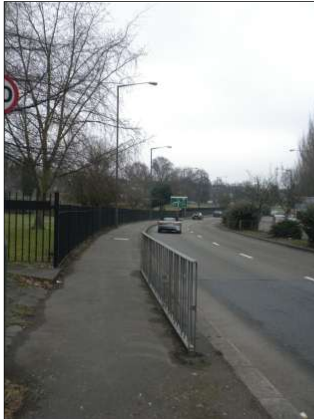
Photo 4 – View of Ring Way part of the AQMA looking south east from Blackwell Street island to Coventry Street island, note open space to the left of the photo.
