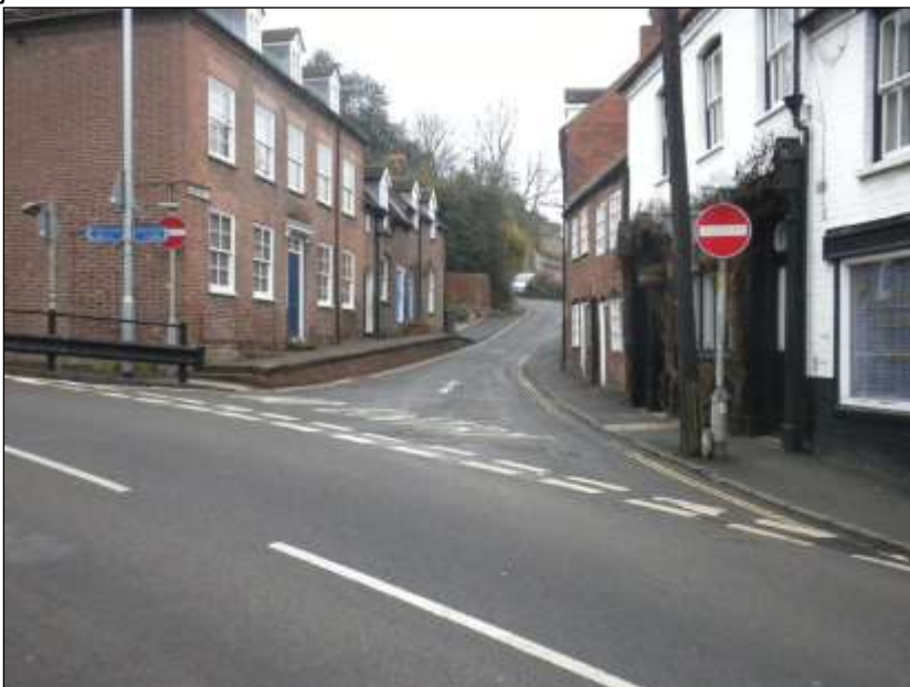
Photo 2 – Looking towards west from the western end of the AQMA to where Richmond Road junctions with Welch Gate
